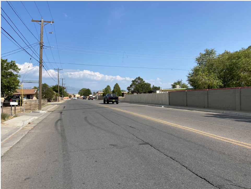
Figure 3: Iliff Road looking East
